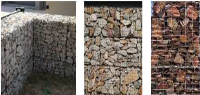
Figure 5: Acceptable stone cladding
